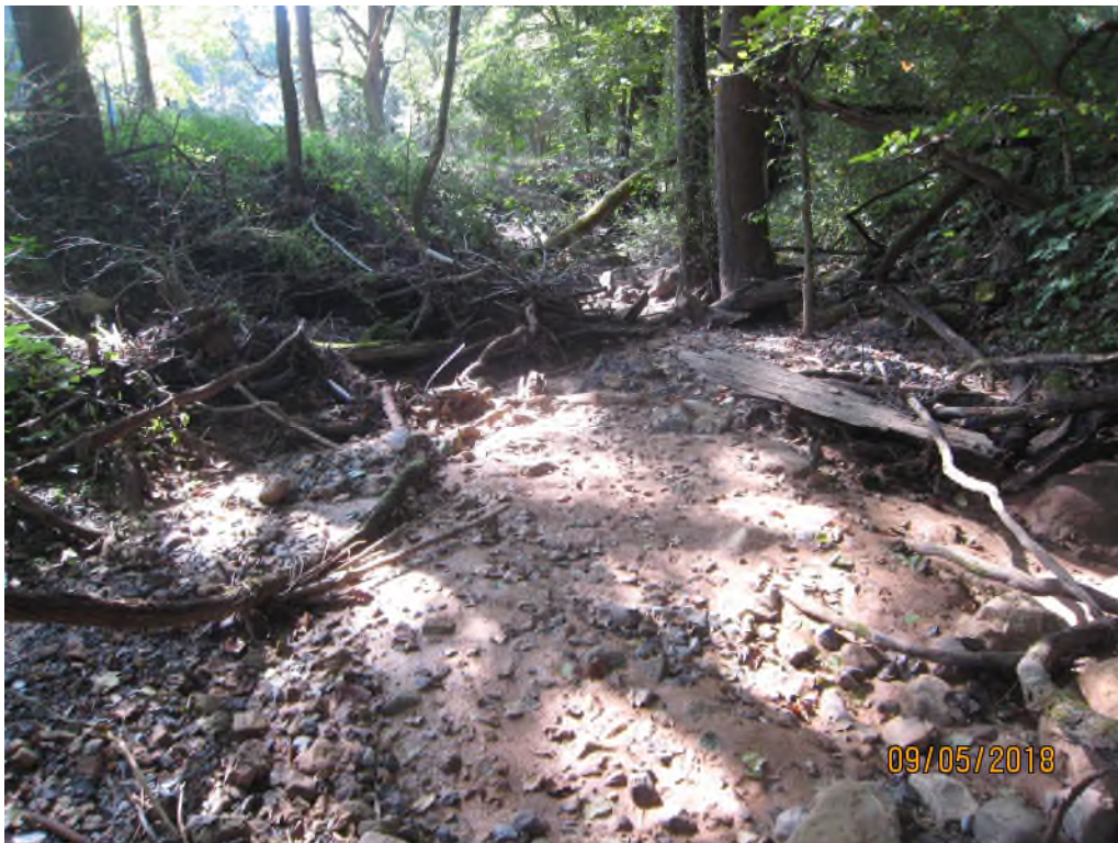
Photo 4: Sediment at debris dam approximately 400' downstream of Photo 1; Depth = 4" Orientation: Downstream
