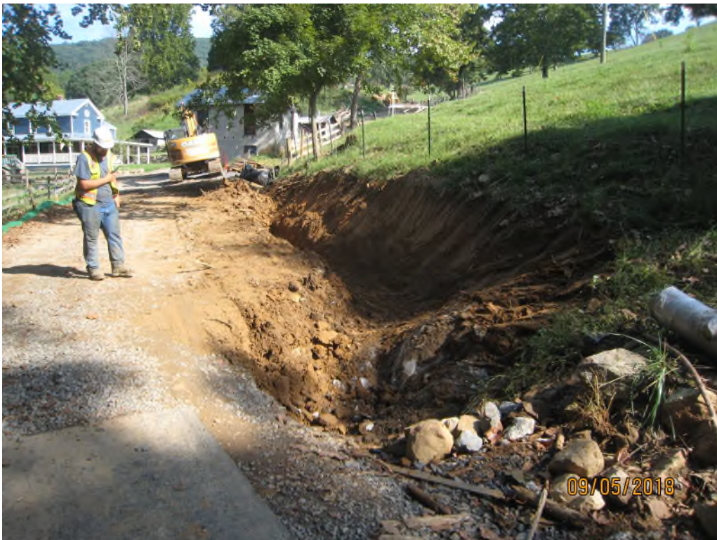
Photo 2: Access Road construction/maintenance near Photo 1 Orientation: Upslope
