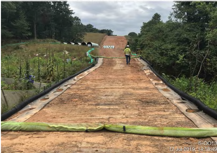
Fig. 3: Stream S-0011 – Controls in place. Bridge clean with functioning sideboards and waddles.
