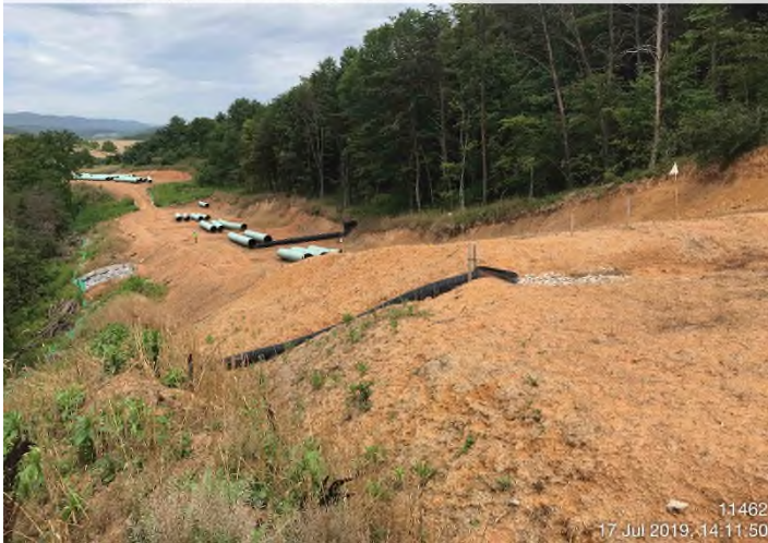
Fig. 3: Stream S-0011 – Controls in place. Bridge clean with functioning sideboards and waddles.
