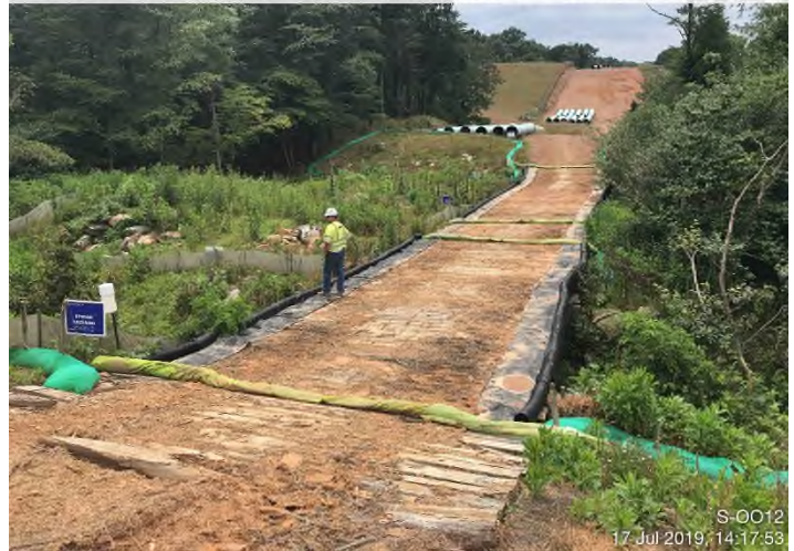
Fig. 4: STA 11432+00 – Sump maintenance needed.
