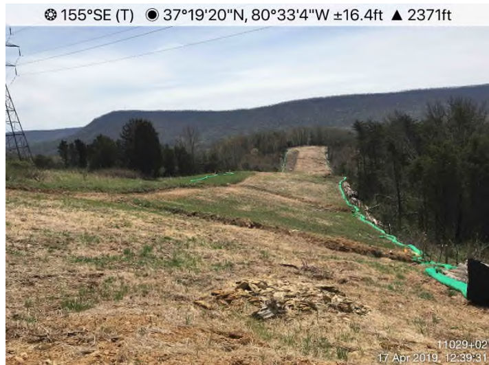
Fig. 8: STA 11029+02 – Area adequately stabilized. Controls in place.
