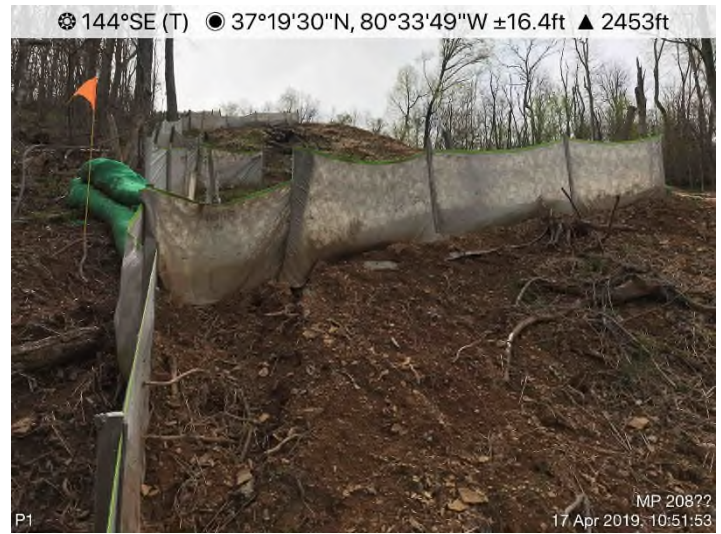
Fig. 4: STA 10991+00 – P1 undermined.
