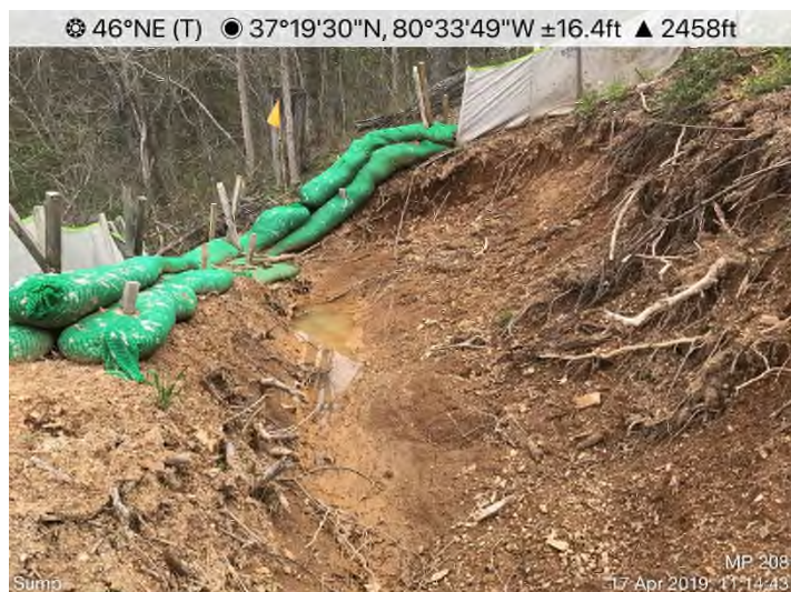
Fig. 7: STA 11025+00 – Area adequately stabilized. Controls in place.
