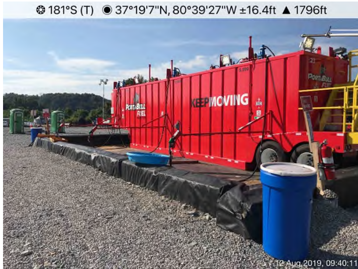
Fig. 3: Laydown Yard 029 – Perimeter controls in place and functioning properly.
