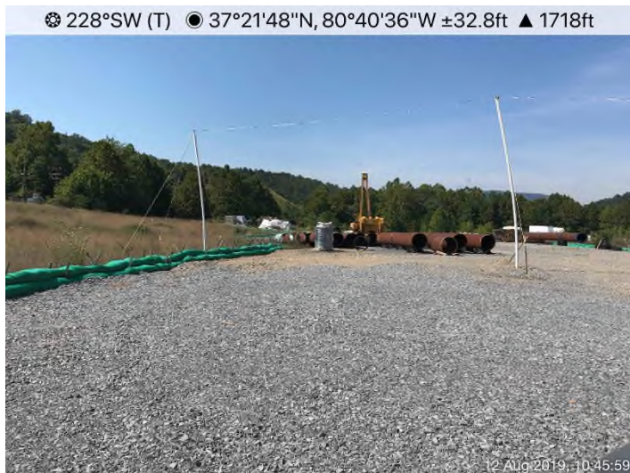
Fig. 3: Laydown Yard 029 – Perimeter controls in place and functioning properly.
