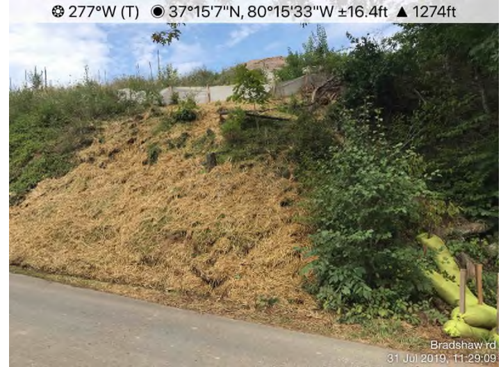
Fig. 4: STA 12190+95 – Bradshaw Road crossing. No evidence of sediment discharge from ROW. Slope stabilized.
