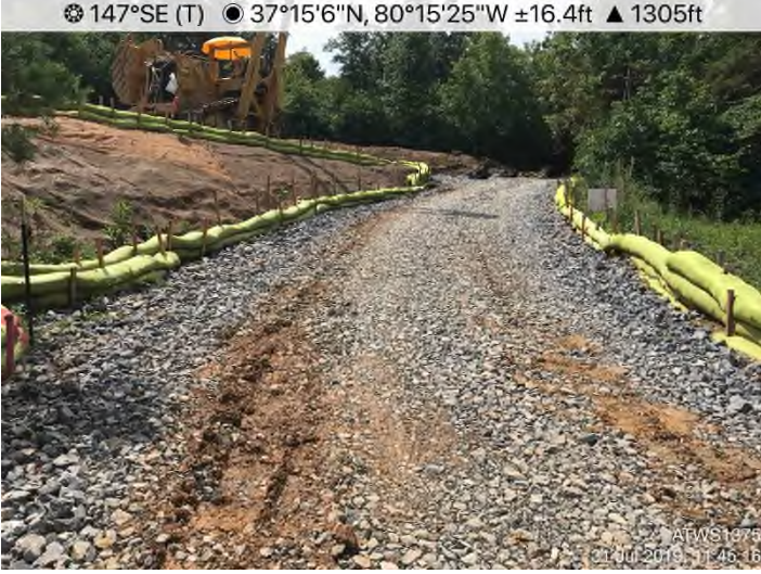
Fig. 19: ATWS 1375 – Controls in place above S-0011 in ATWS 1375. Stone is clean and perimeter controls in place and functioning.
