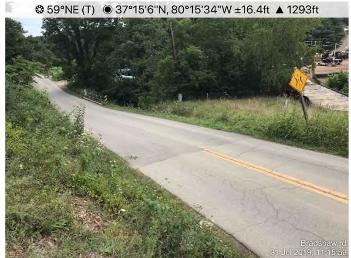
Fig. 4: STA 12190+95 – Bradshaw Road crossing. No evidence of sediment discharge from ROW. Slope stabilized.
