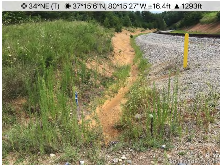
Fig. 15: MVP-MN-275 – RVRA east track swale leading to S-OO11 south side of access road MVP-MN-275. Sediment accumulation evident in culvert and swale.
