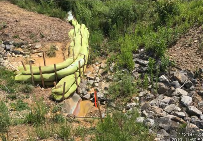
Fig. 19: ATWS 1375 – Controls in place above S-0011 in ATWS 1375. Stone is clean and perimeter controls in place and functioning.
