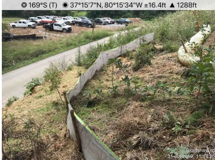
Fig. 3: STA 12190+75 – Bradshaw Road crossing. No evidence of sediment discharge from ROW. Controls functioning and area stabilized.
