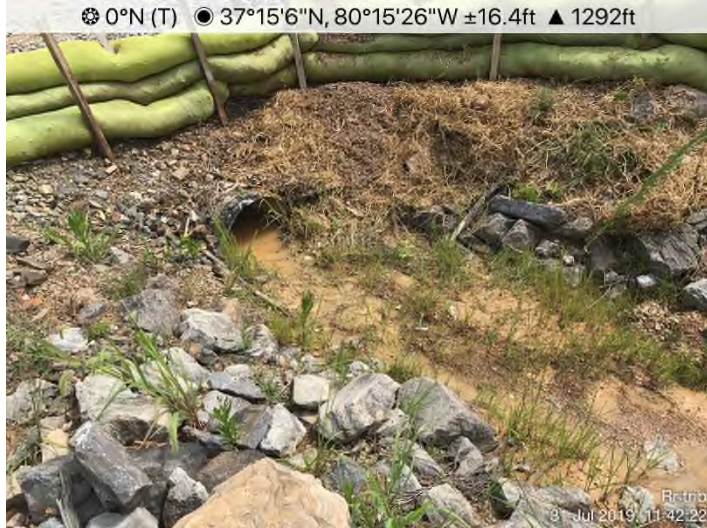
Fig. 15: MVP-MN-275 – RVRA east track swale leading to S-OO11 south side of access road MVP-MN-275. Sediment accumulation evident in culvert and swale.
