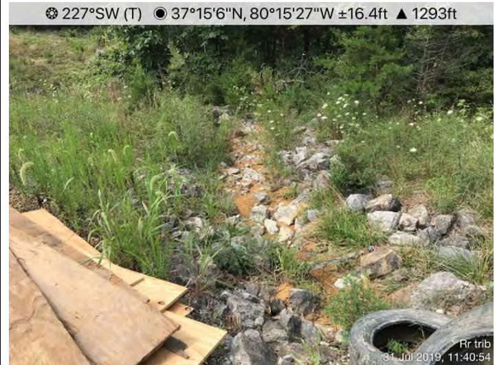
Fig. 16: MVP-MN-275 – Sediment accumulation in RVRA east track swale leading to S-OO11 south side of access road MVP-MN-275.
