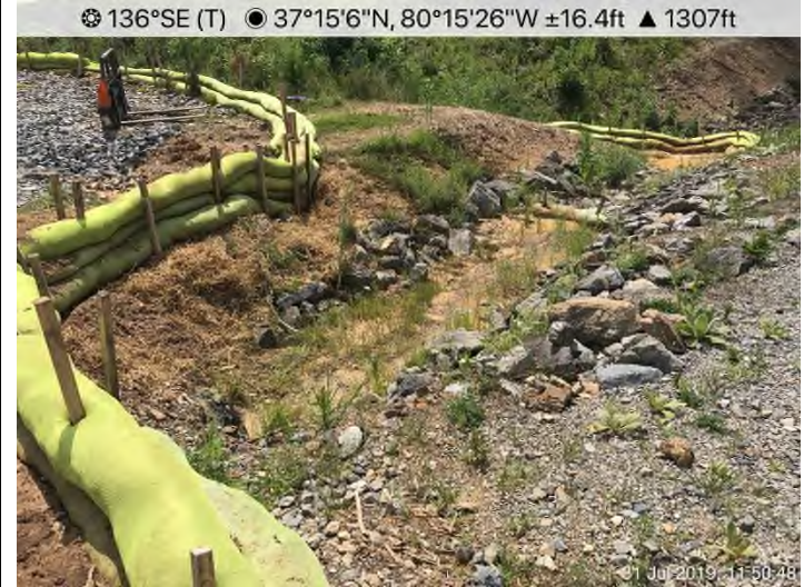
Fig. 16: MVP-MN-275 – Sediment accumulation in RVRA east track swale leading to S-OO11 south side of access road MVP-MN-275.
