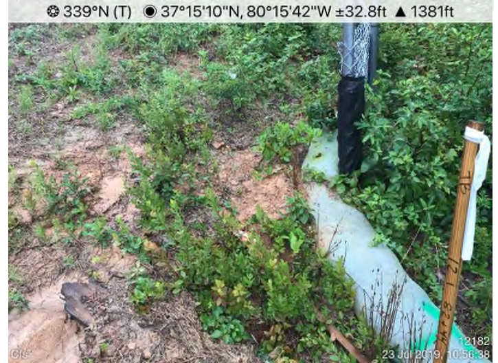
Fig. 4: STA 12182+44 – CFS maintenance needed.
