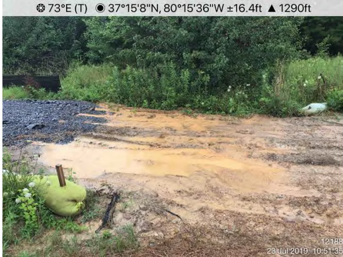
Fig. 3: STA 12188+00 – ECDs needed between AEP entrance and MVP ROW.
