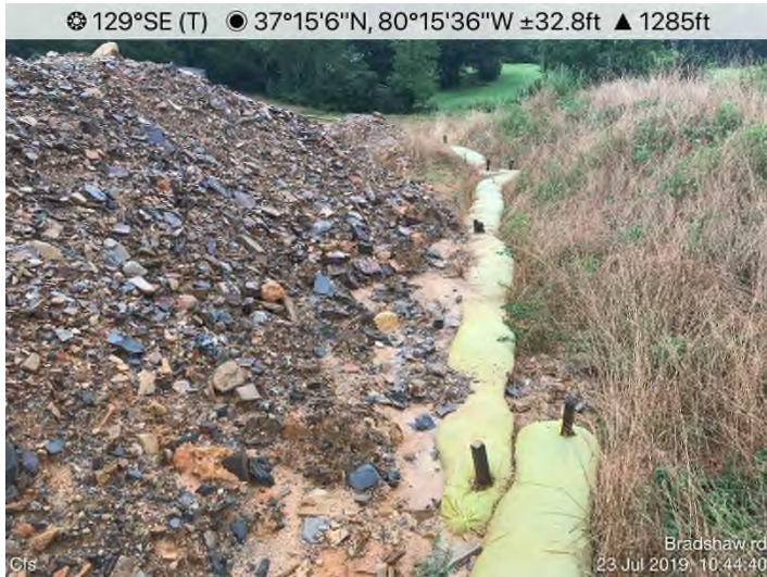
Fig. 3: STA 12188+00 – ECDs needed between AEP entrance and MVP ROW.
