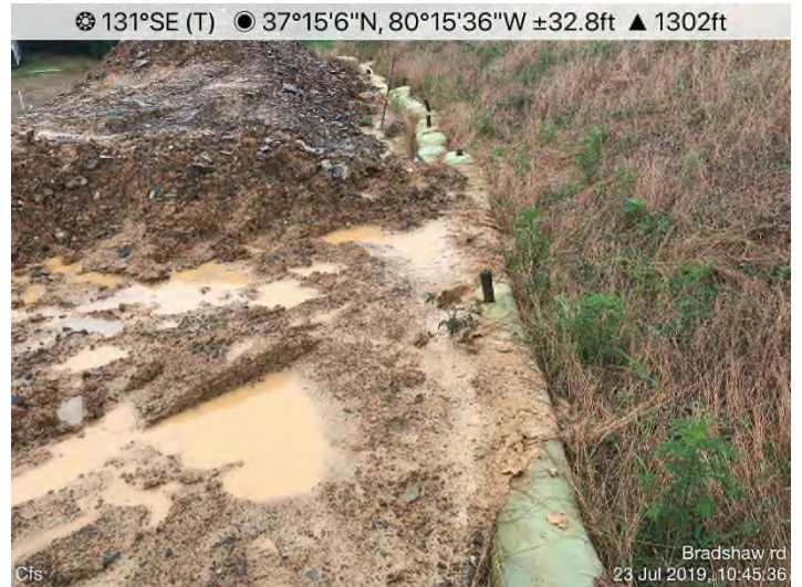
Fig. 4: STA 12182+44 – CFS maintenance needed.
