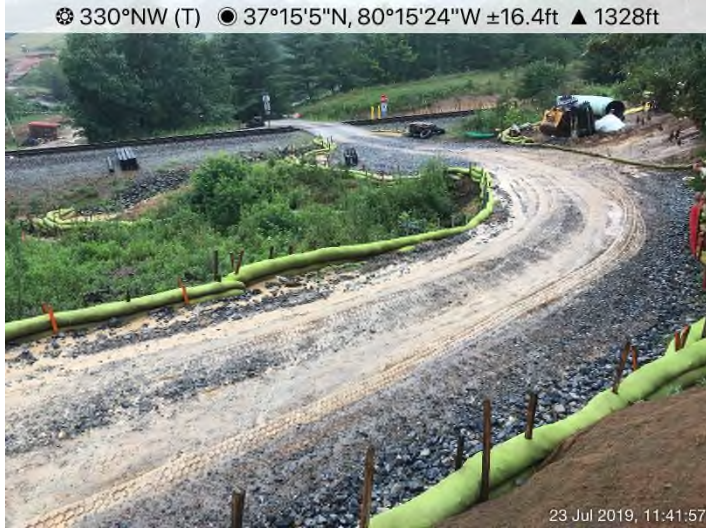
Fig. 11: ATWS 1375 – Looking NW from ATWS 1375 towards stream S-OO11. Stone needs refreshing/top-dressing.
