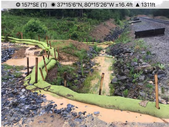
Fig. 11: ATWS 1375 – Looking NW from ATWS 1375 towards stream S-OO11. Stone needs refreshing/top-dressing.
