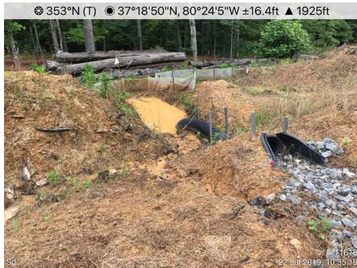
Fig. 3: STA 11901+00 – CFS maintenance needed.
