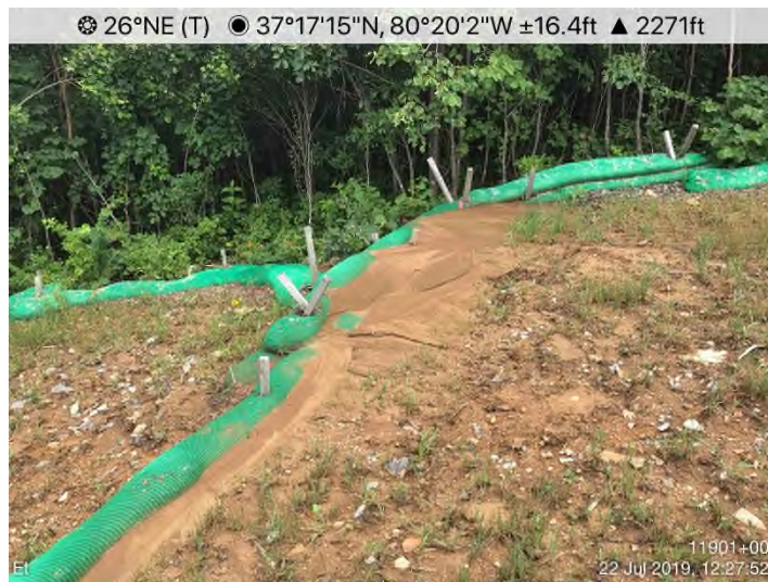
Fig. 3: STA 11901+00 – CFS maintenance needed.
