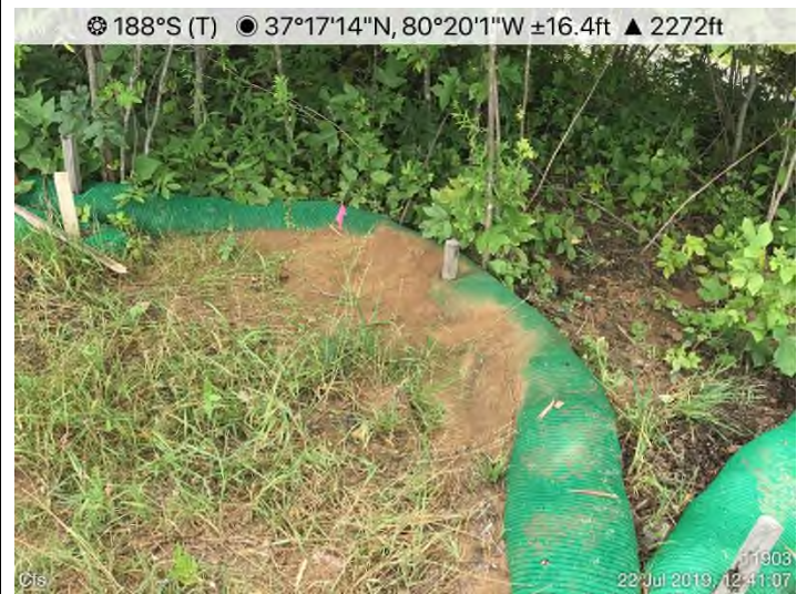
Fig. 4: STA 11903+00 – CFS maintenance needed.
