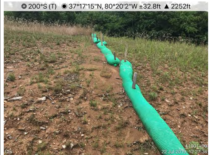
Fig. 4: STA 11903+00 – CFS maintenance needed.
