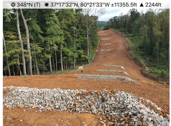
Fig. 4: STA 11886+00 – Final restoration completed. Controls in place and functioning. Area stabilized with straw, seed and erosion fabric.
