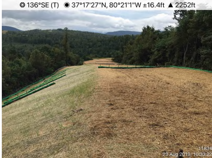
Fig. 3: STA 11834+00 – Final restoration completed. Controls in place and functioning. Area stabilized with straw, seed and erosion fabric.
