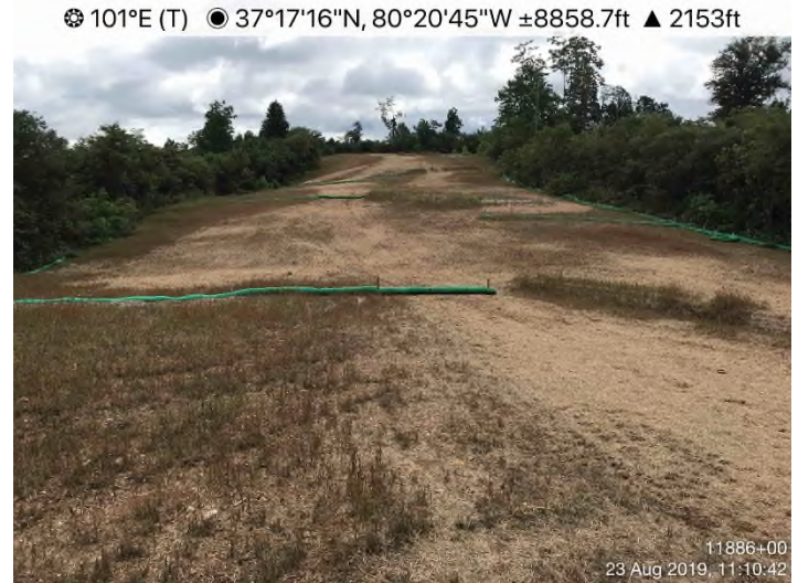
Fig. 4: STA 11886+00 – Final restoration completed. Controls in place and functioning. Area stabilized with straw, seed and erosion fabric.
