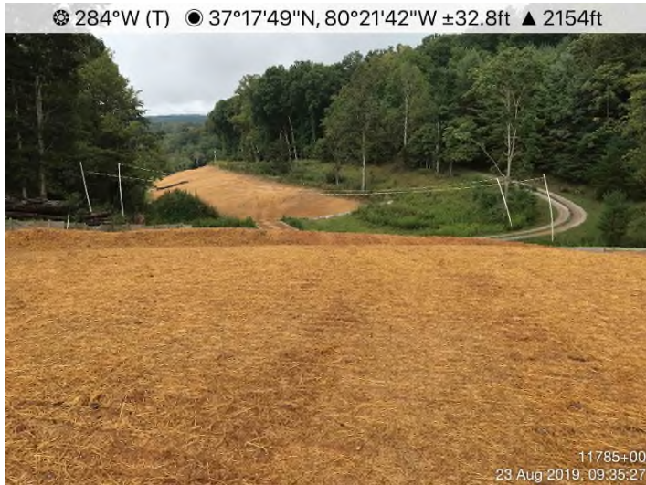
Fig. 3: STA 11834+00 – Final restoration completed. Controls in place and functioning. Area stabilized with straw, seed and erosion fabric.
