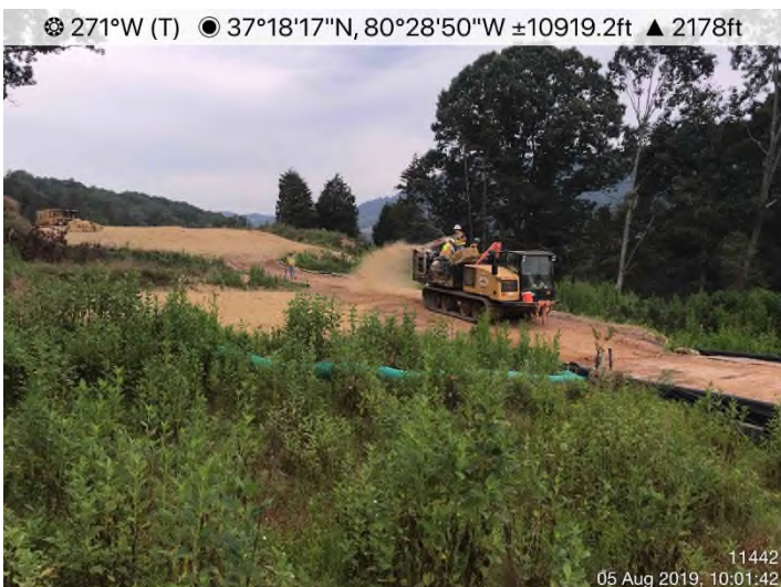
Fig. 3: STA 11442+00 – Controls in place. Active re-stabilization efforts of straw and millet.
