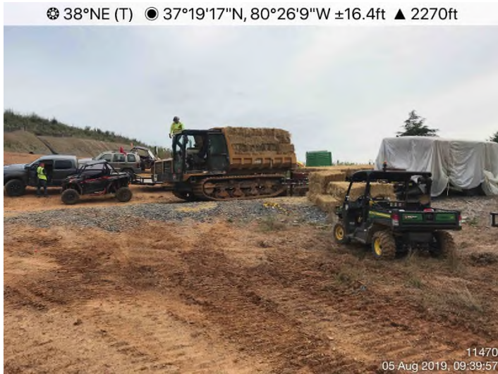
Fig. 3: STA 11442+00 – Controls in place. Active re-stabilization efforts of straw and millet.
