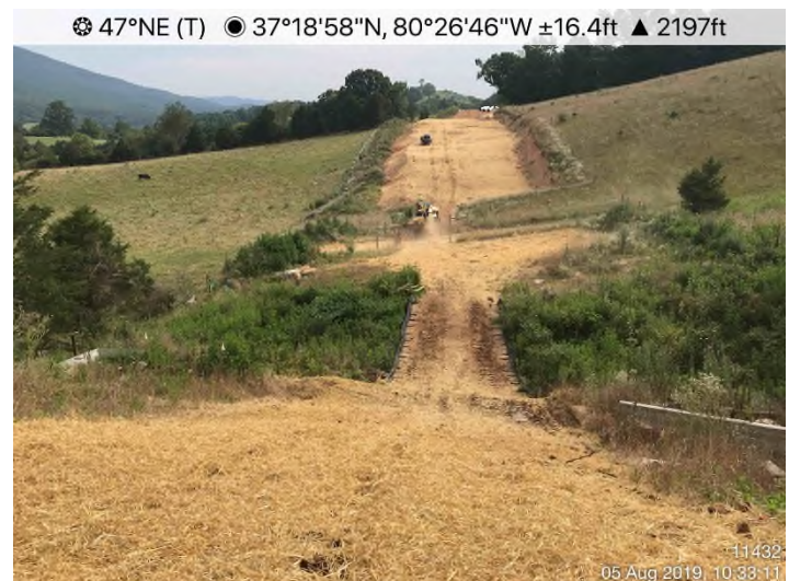
Fig. 4: STA 11432+00 – Controls in place. Area re-stabilized with millet and straw.
