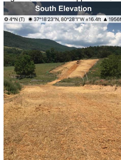
Fig. 4. Stabilization applied at St11354
