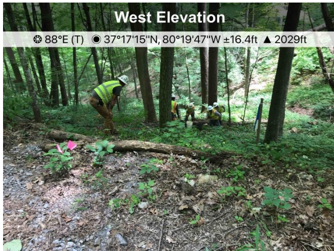
Fig. 3. Repairs and offsite gravel removal being conducted on AR 266.03
