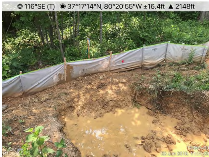
Fig. 7: STA 11901+00 – Maintain/cleanout CFS.
