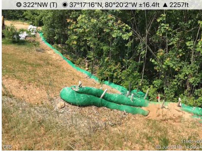
Fig. 7: STA 11901+00 – Maintain/cleanout CFS.
