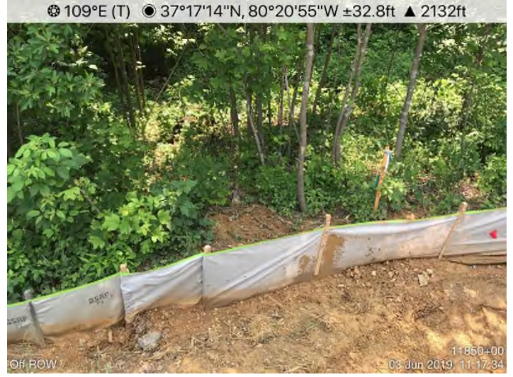
Fig. 8: STA 11889+00 – Maintain/cleanout CFS.
