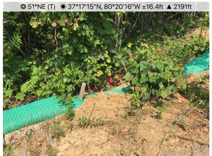
Fig. 8: STA 11889+00 – Maintain/cleanout CFS.
