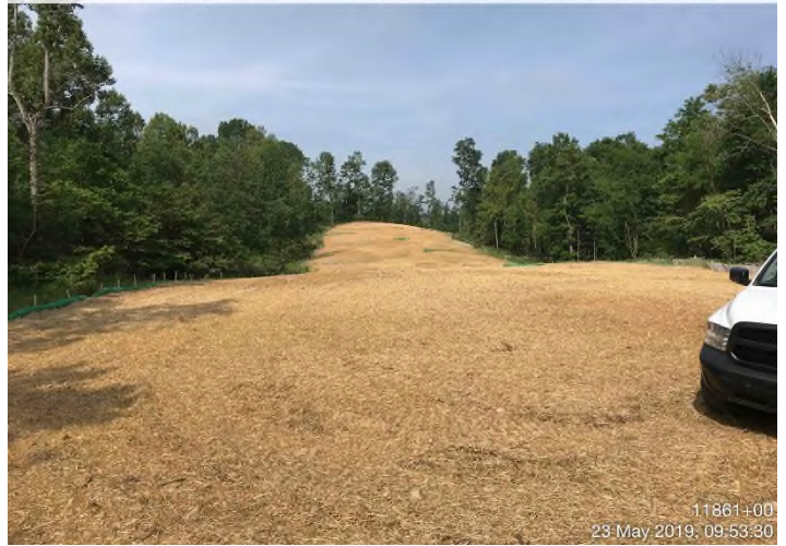
Fig. 4: STA 11885+00 – Controls in place. Topsoil disked.
