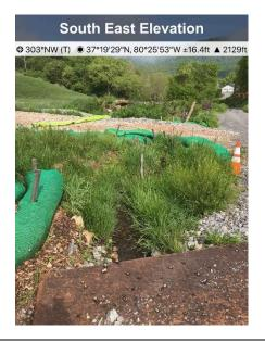
Fig. 3 Above designated streams S-0012 and S-0013, ECD's in place.
