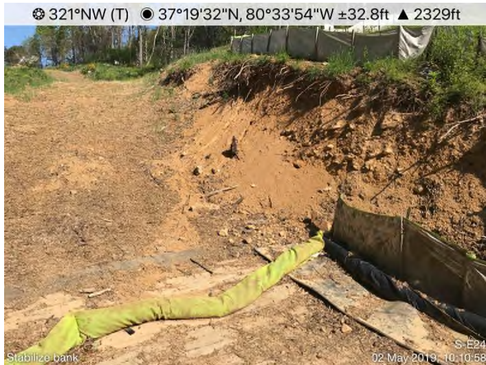
Fig. 3: STA 10985+50 – Stabilize erosion CIS stream S-E24.
