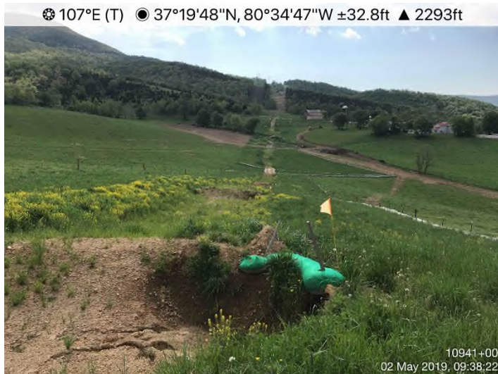
Fig. 3: STA 10985+50 – Stabilize erosion CIS stream S-E24.
