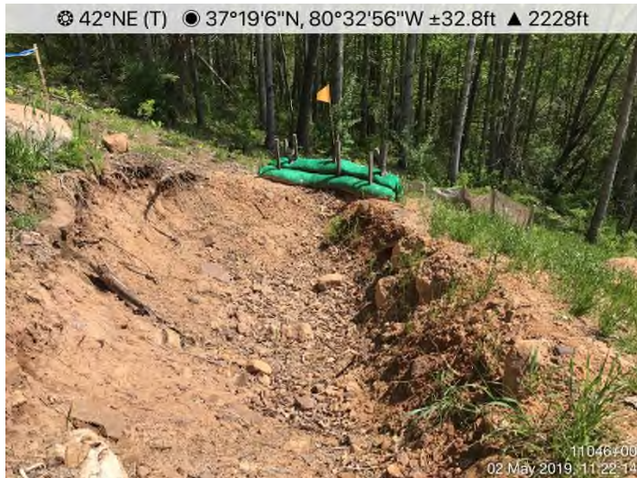
Fig. 7: STA 11120+00 – Waterbar maintenance needed.
