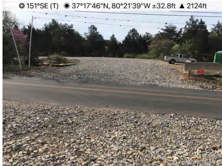
Fig. 3: STA 11788+06 – RCE at Mt. Tabor Road adequately maintained.
