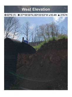
Fig. 4 St#11473 two tone area is eroding and requires repair / stabilization
