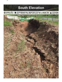
Fig. 2 St#11511+00 two tone area is eroding and requires repair / stabilization
