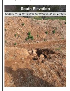
Fig. 3 St#11489 clean water diversion inlet has eroded
