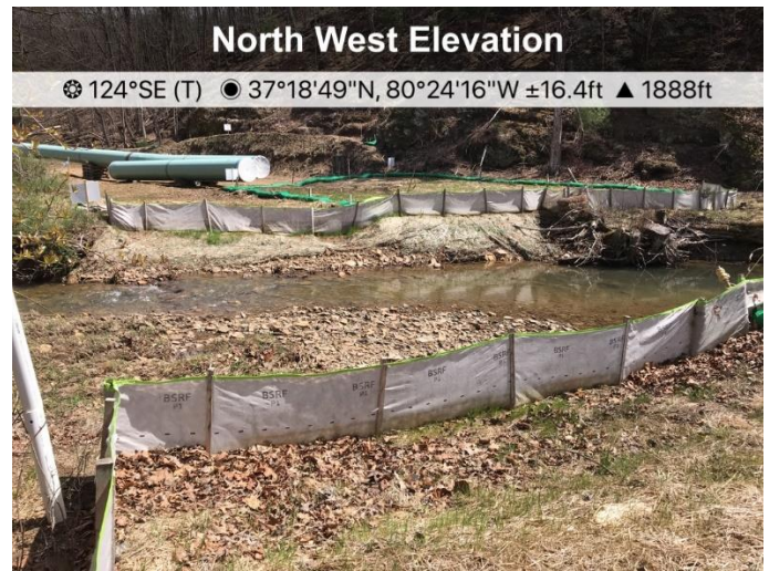
Fig. 4 Designated stream S-006, ECD's in place
