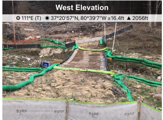
Fig. 2 Designated stream S-G32, ECD's in place
