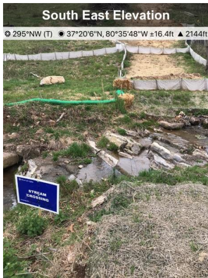
Fig. 3 Designated stream S-A32, ECD's in place
