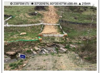
Fig. 3: **STA 10906+00** – Area adequately stabilized. Controls in place.
