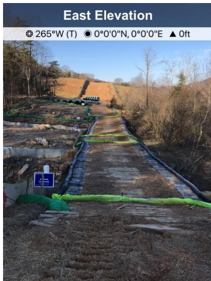
Fig. 3 Near streams S-0012 ECD's are in place and functioning
