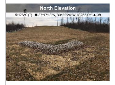
Fig. 2 At karsts feature 226.42, ECD's are in place and functioning
