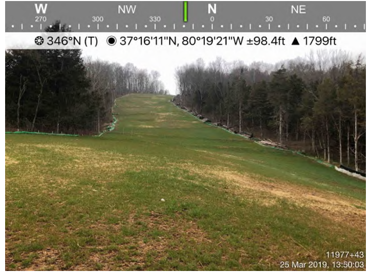
Fig. 8: STA 11977+43 – Area adequately stabilized. Controls in place.
