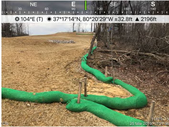
Fig. 7: STA 11879+16 – Clean out CFS. Repair/stabilize erosion.
