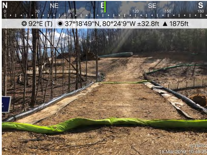
Fig. 3: STA 11606+00 – Area adequately stabilized. Controls in place.
