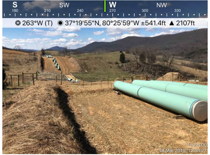
Fig. 8: STA 11501+11 – Area adequately stabilized. Controls in place.
