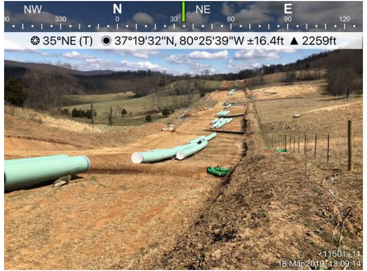
Fig. 8: STA 11501+11 – Area adequately stabilized. Controls in place.
