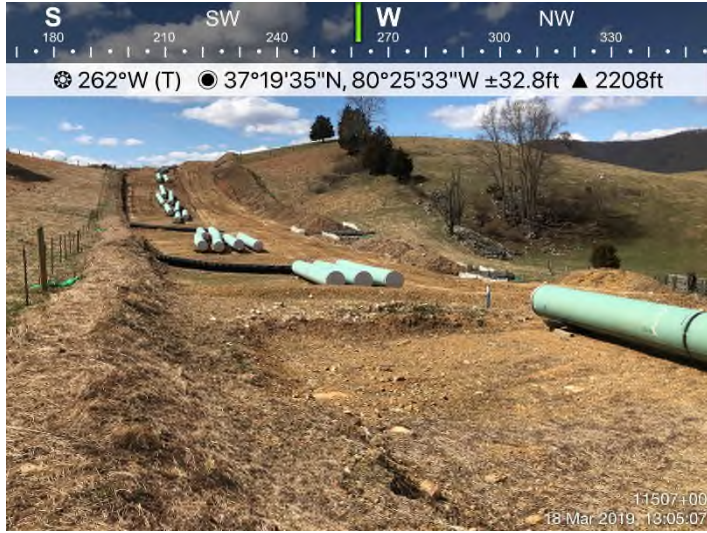
Fig. 7: STA 11507+00 – Area adequately stabilized. Controls in place.
