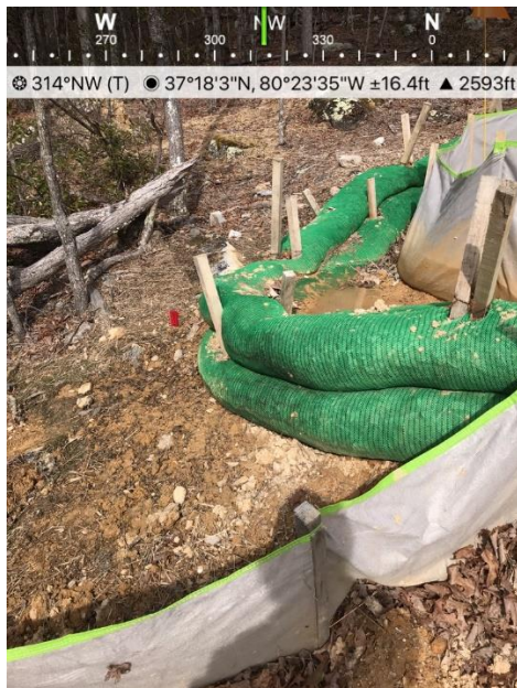
Fig. 3 St#11679+40 sump triple stack is undermined
