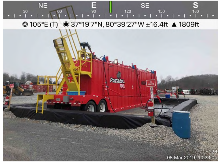
Fig. 4: LY 026 – Secondary containment in place and functioning.
