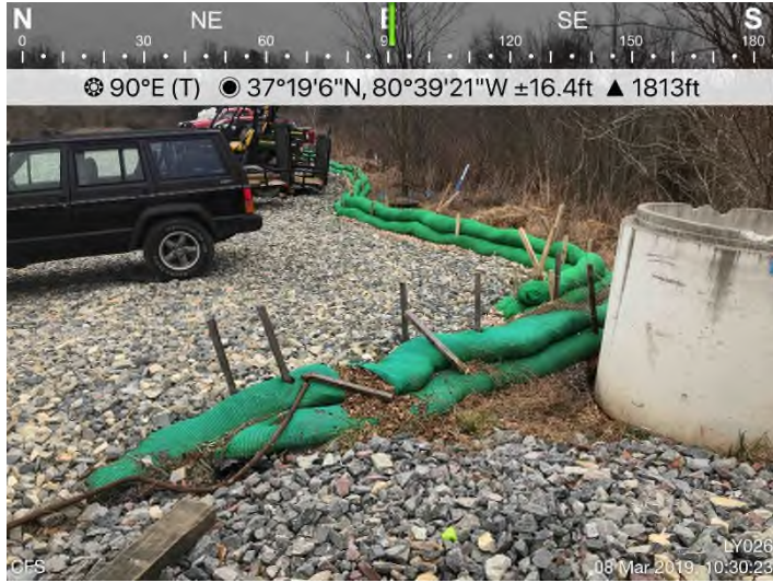
Fig. 3: LY 026 – CFS needs maintenance.
