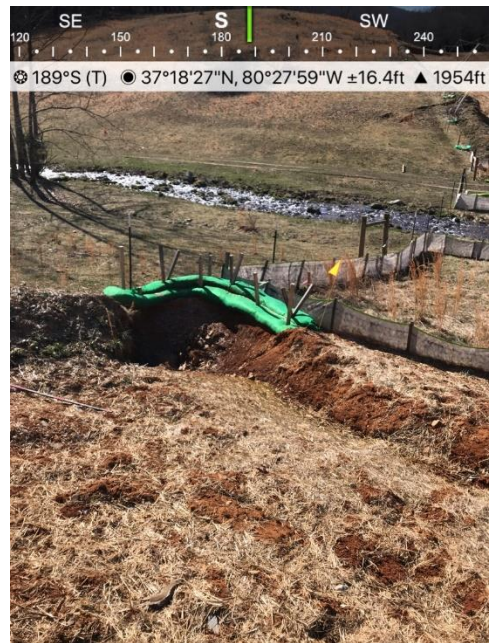
Fig. 4 St#11361+00 sump end treatment is undermined
