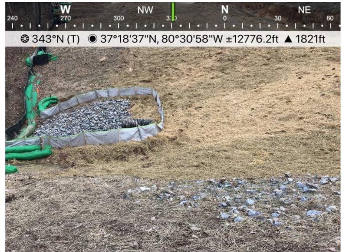
Fig. 2 ST#11184+00 plunge pool area has been repaired
