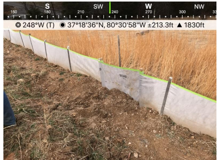
Fig. 4 At St#11172+48 P1 control has been repaired.
