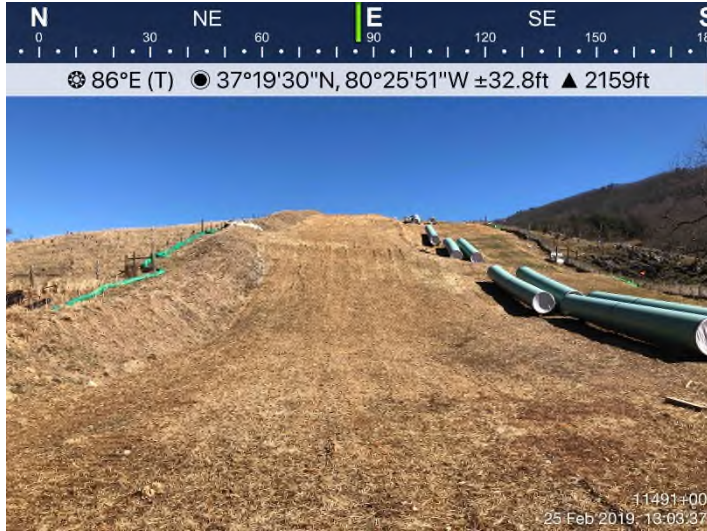
Fig. 3: STA 11491+00 – Area stabilized. Controls in place.
