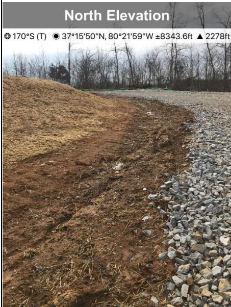
Fig. 3 AR GI234 rock lined channel requires maintenance
