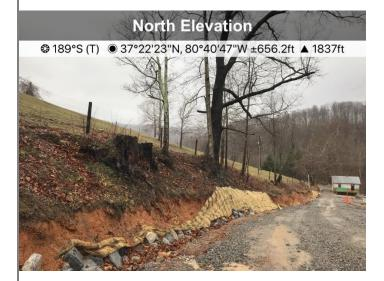
Fig. 2 Near St#11932+54 ECD's in place and functioning
