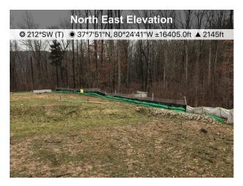
Fig. 4 St#11961+00 ECD's in place and functioning
