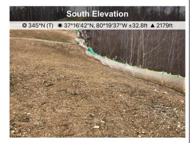
Fig. 3 Near St#11961 area lacks adequate stabilization
