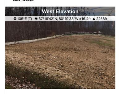
Fig. 2 Near St#11942 area lacks adequate stabilization
