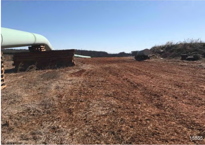
Figure 3: STA 15874+00 – Controls in place and functioning properly. Area stabilized with straw. No erosion evident.
