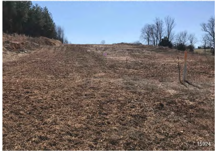
Figure 8: STA 15924+00 – Controls in place and functioning properly. Area stabilized with straw. No erosion evident. BRG: 152°SE (T) LAT: 36.840938 LON: -79.366688 ±16ft ALT: 620ft
