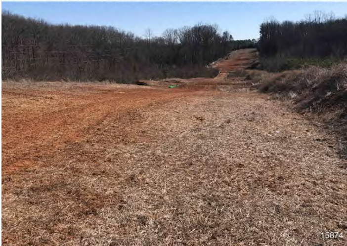
Figure 3: STA 15874+00 – Controls in place and functioning properly. Area stabilized with straw. No erosion evident.
