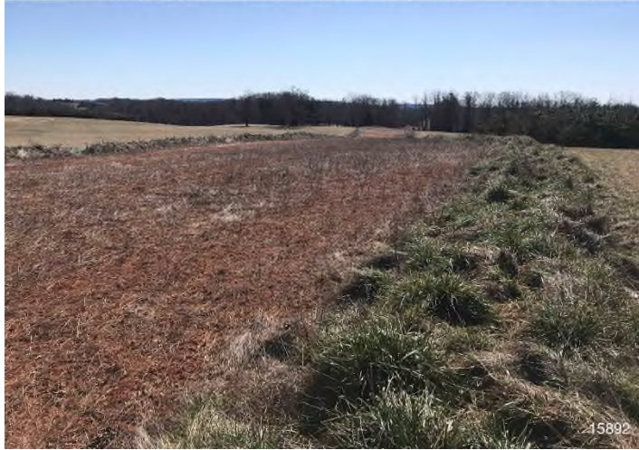
Figure 7: STA 15920+00 – Controls in place and functioning properly. Area stabilized with straw. No erosion evident. BRG: 158°S (T) LAT: 36.841984 LON: -79.367466 ±16ft ALT: 639ft
