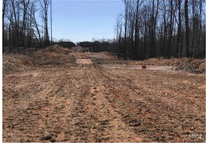
Figure 8: STA 15924+00 – Controls in place and functioning properly. Area stabilized with straw. No erosion evident. BRG: 152°SE (T) LAT: 36.840938 LON: -79.366688 ±16ft ALT: 620ft
