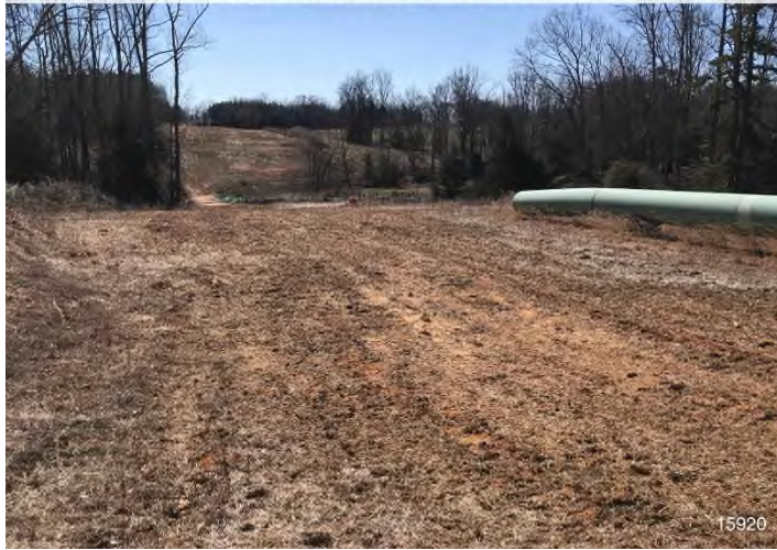
Figure 7: STA 15920+00 – Controls in place and functioning properly. Area stabilized with straw. No erosion evident. BRG: 158°S (T) LAT: 36.841984 LON: -79.367466 ±16ft ALT: 639ft
