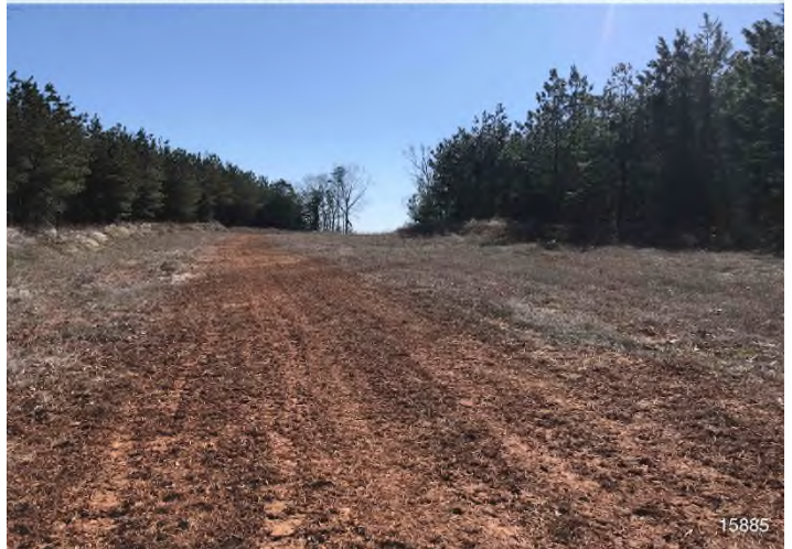
Figure 4: STA 15885+00 – Controls in place and functioning properly. Area stabilized with straw. No erosion evident.
