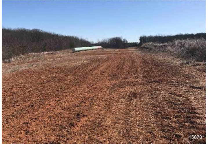
Figure 4: STA 15885+00 – Controls in place and functioning properly. Area stabilized with straw. No erosion evident.
