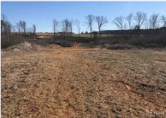
Figure 7: STA 15444+00 – Controls in place and functioning properly. Area stabilized with straw. No erosion evident.
