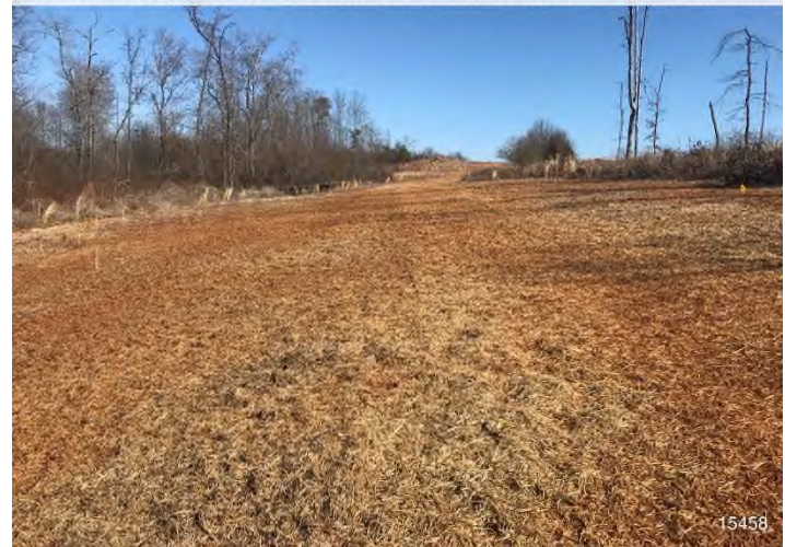
Figure 8: STA 15458+00 – Controls in place and functioning properly. Area stabilized with straw. No erosion evident.
