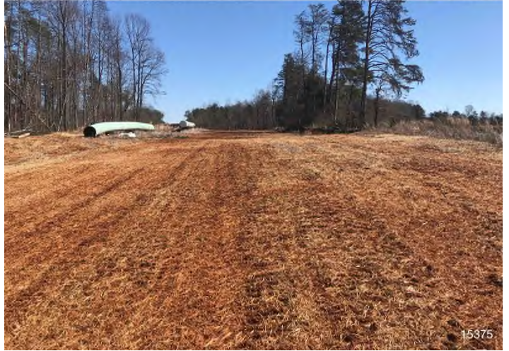
Figure 4: STA 15416+00 – Controls in place and functioning properly. Area stabilized with straw. No erosion evident.
