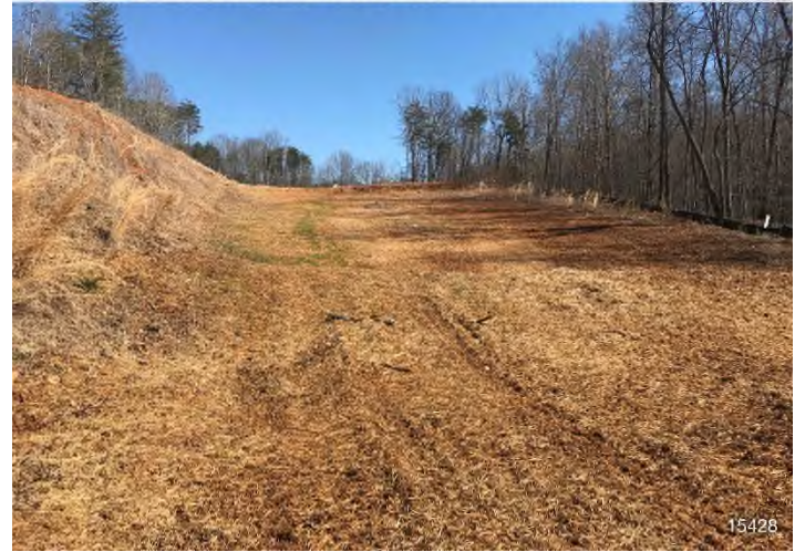
Figure 8: STA 15458+00 – Controls in place and functioning properly. Area stabilized with straw. No erosion evident.
