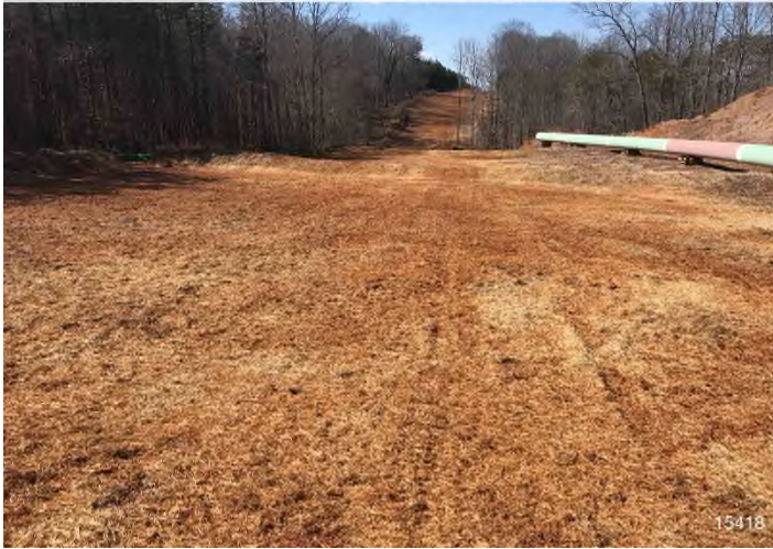
Figure 7: STA 15444+00 – Controls in place and functioning properly. Area stabilized with straw. No erosion evident.
