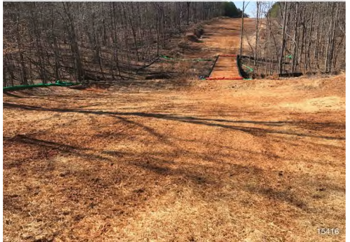
Figure 4: STA 15416+00 – Controls in place and functioning properly. Area stabilized with straw. No erosion evident.
