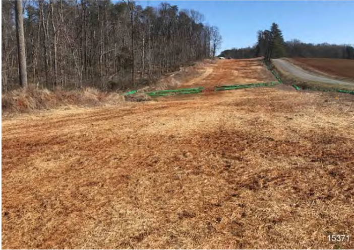
Figure 3: STA 15405+00 – Controls in place and functioning properly. Area stabilized with straw. No erosion evident.
