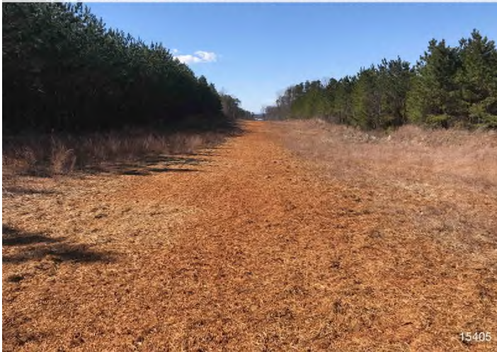
Figure 3: STA 15405+00 – Controls in place and functioning properly. Area stabilized with straw. No erosion evident.
