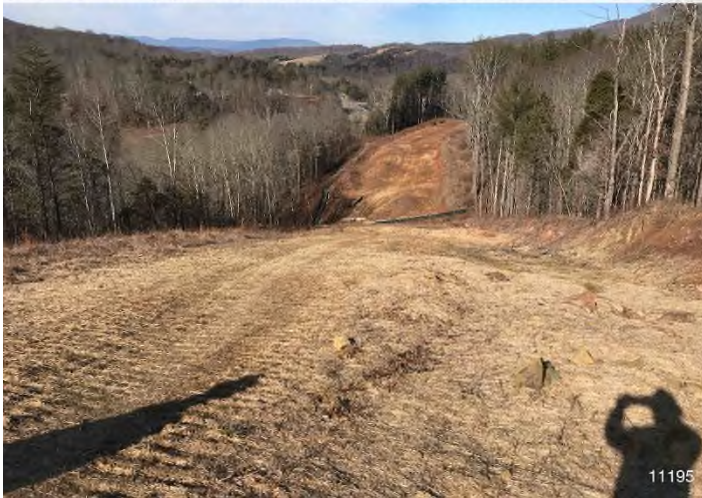
Figure 3: STA 11195+00 – Controls in place and functioning properly. Area stabilized with straw.
