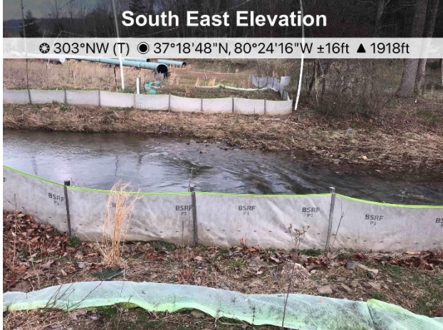
Figure 3: Designated crossing S-RR006, ECD's are in place.
