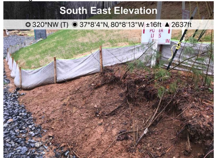
Figure 4: Additional stabilization requires on denuded slope along AR RO 287.
