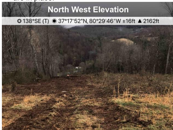
Figure 3: Near St11248+00 area is planned for grubbing, ECD's are in place.
