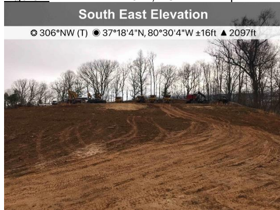
Figure 1: Near ATWS 1347, ECD's are in place.
