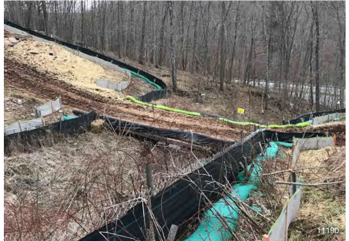
Figure 4: STA 11190+00 – Controls in place and functioning properly. BRG: 169°S (T) LAT: 37.306290 LON: -80.509893 ±32ft ALT: 1947ft
