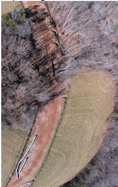
Photo 3. MVW Photo Jan. 14, 2021 at MP 302.1 showing alleged inadequate vegetative stabilization.
