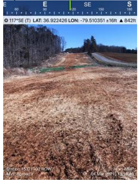
Photo 2. MBP Photo Mar. 4, 2021 near MP 291 showing temporary stabilization with straw. Note straw is stained by red soil.
