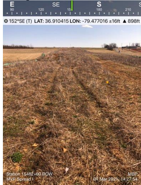
Photo 6. MBP Photo Mar.4, 2021 near MP 293.1 showing adequate vegetative stabilization.
