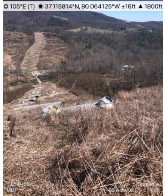
Photo 13. MBP photo from April 2, 2021 showing land-disturbance outside the ROW from logging and 4-wheel drive activities.
