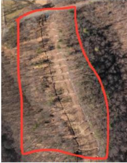
Milepost 249.9 G0020965 Inspection requested for evidence of sediment off the left side of ROW.
