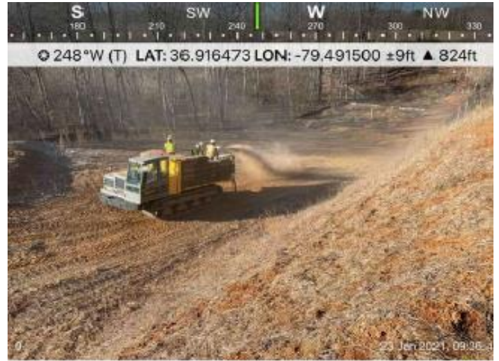
Photo 6. MVP photo showing hydraulic application of seed.
