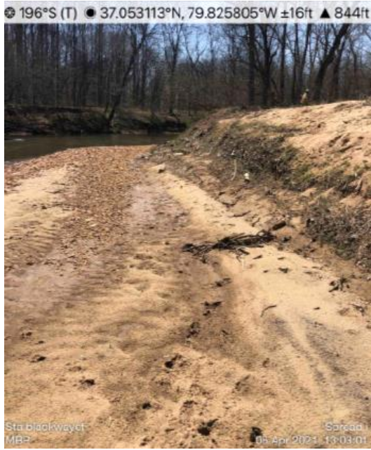
Photo 11. MVW photo soil slip. MVP has stabilized this area and is currently working on a plan to remedy the slip.
