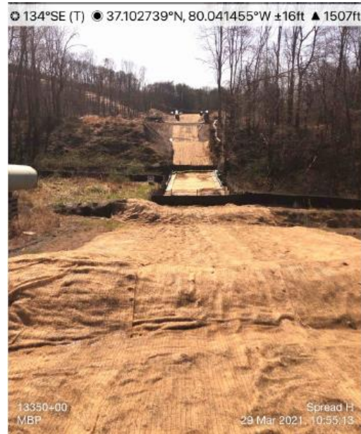
Photo 4. MBP photo showing blankets and matting providing temporary soil stabilization.
