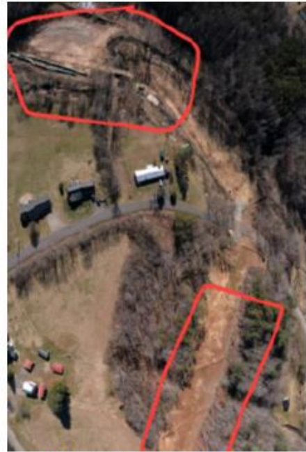
Milepost 260.2 G0020665 Inspection requested for sparsely vegetated areas.
