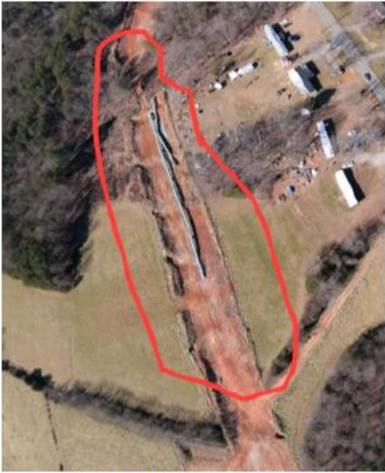
Milepost 271.4 G0020328 Inspection requested for sparsely vegetated area. Reseeding needed.
