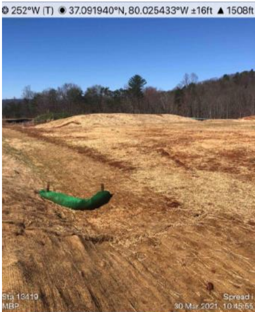
Photo 3. MBP photo showing straw providing temporary soil stabilization.
