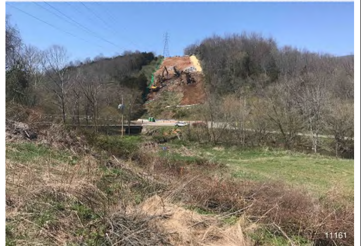
Figure 4: STA 11161+00 – Controls in place and functioning properly. BRG: 299°NW (T) LAT: 37.310801 LON: -80.515844 ±541ft ALT: 1832ft
