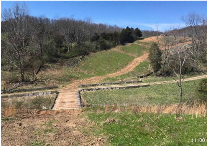
Figure 3: STA 11100+00 – Controls in place and functioning properly. BRG: 273°W (T) LAT: 37.313195 LON: -80.533283 ±32ft ALT: 1984ft
