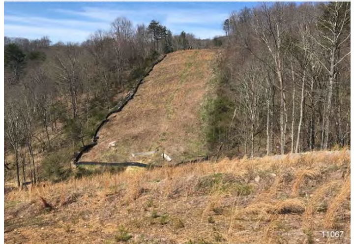
Figure 4: STA 11067+00 – Controls in place and functioning properly. BRG: 92°E (T) LAT: 37.306213 LON: -80.508641 ±13639ft ALT: 2168ft
