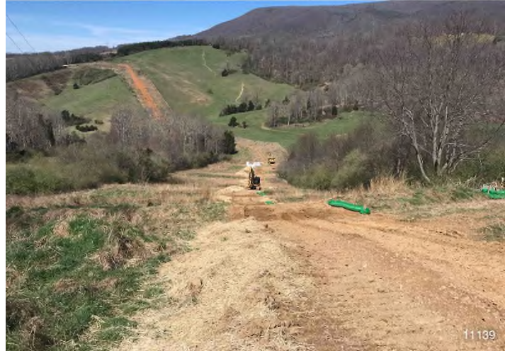
Figure 2: STA 11139+00 – Controls in place and functioning properly. BRG: 305°NW (T) LAT: 37.313599 LON: -80.522308 ±16ft ALT: 2149ft
