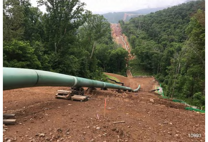
Figure 2: STA 10993+00 – Controls in place and functioning properly. BRG: 311°NW (T) LAT: 37.324776 LON: -80.562949 ±16ft ALT: 2587ft
