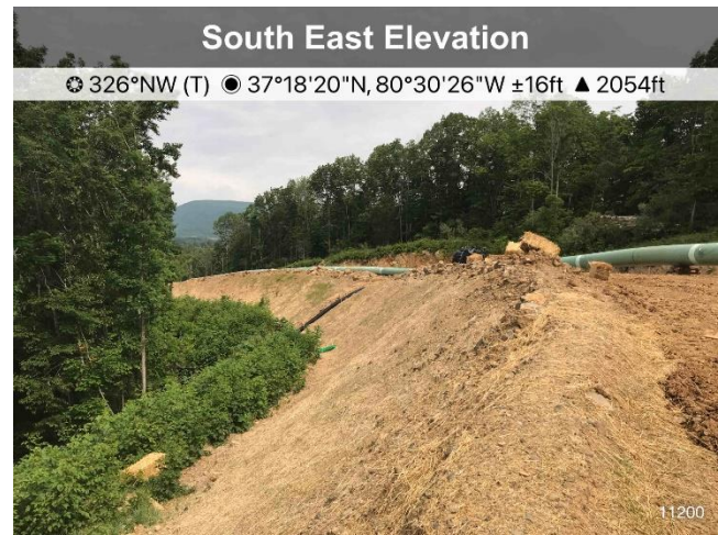
Figure 4: St 11200 stabilized slope
