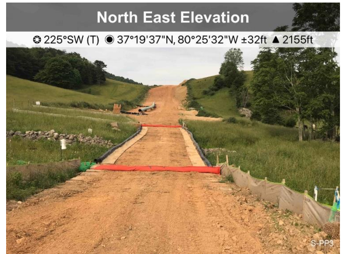
Figure 2: Designated crossing S-PP3, ECD's are in place.
