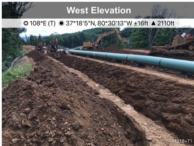
Figure 3: St11218+71 active trenching
