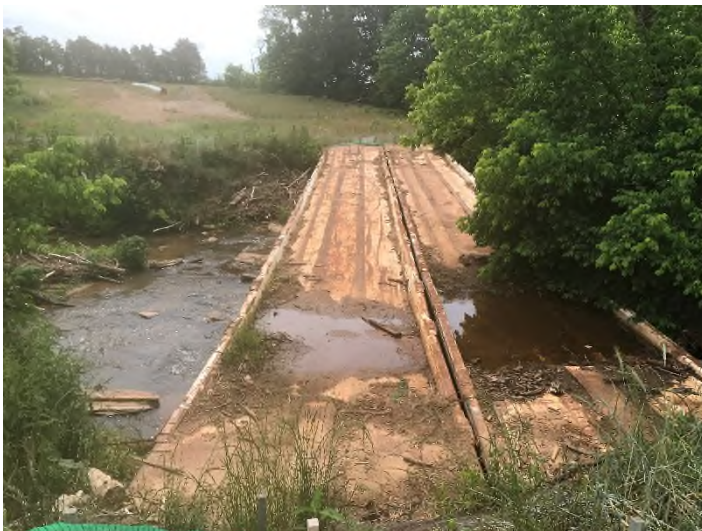
Figure 3: Stream S-II2 (Little Creek) – MVP temporary equipment crossing. Bridge does not impede normal flow conditions.
