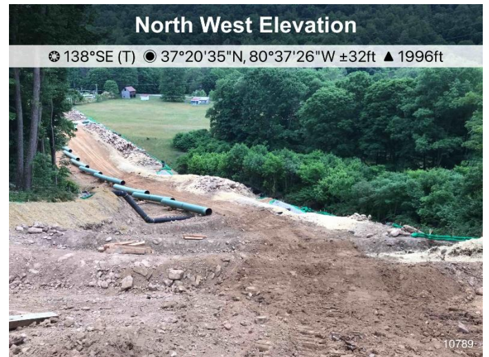
Figure 4: ECD's are in place and pipe is strung near St10789.
