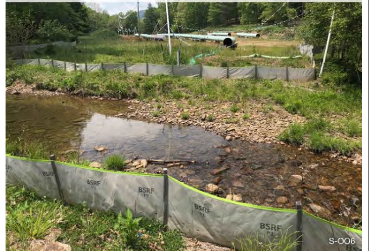
Figure 4: Stream S-006 – Controls in place and functioning properly around Craig Creek. BRG: 261°W (T) LAT: 37.313637 LON: -80.404490 ±16ft ALT: 1901ft
