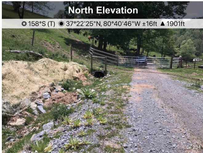
Figure 1: Access road GI 234 matting remains installed.
