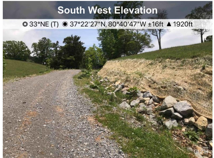
Figure 2: Access road GI 234 matting remains installed.
