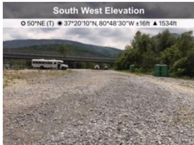
Figure 4: Pollution prevention devices in place at Yard 28.
