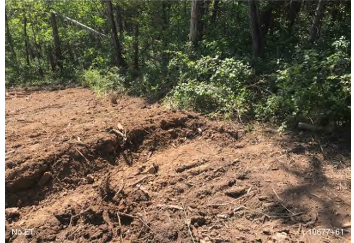
Figure 2: STA 10677+61 – Topsoil waterbar does not have end-treatment.
