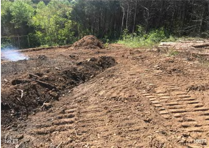
Figure 1: STA 10677+00 – Topsoil waterbar does not have end-treatment.
