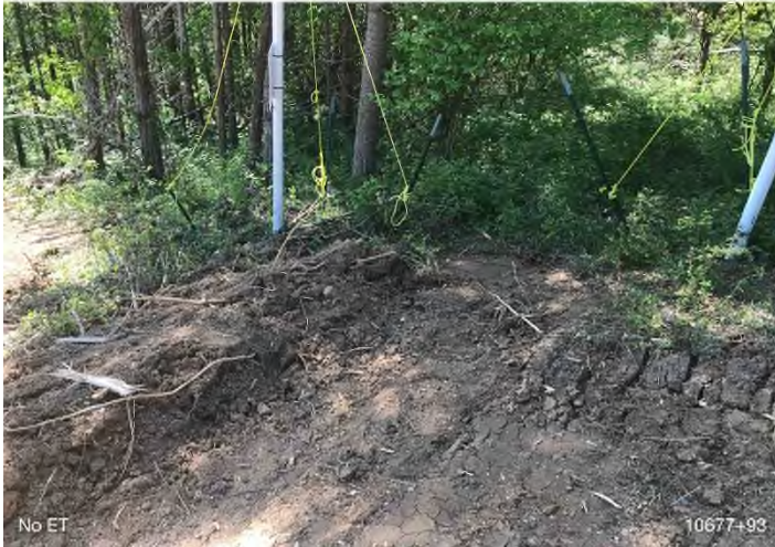
Figure 3: STA 10677+93 – Topsoil waterbar does not have end-treatment.
