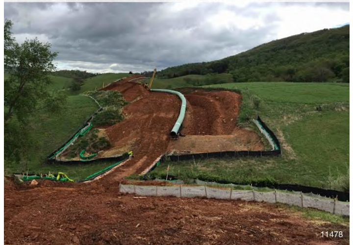
Figure 4: STA 11478+00 – Controls in place and functioning properly. BRG: 65°NE (T) LAT: 37.280701 LON: -80.388092 ±6562ft ALT: 2148ft
