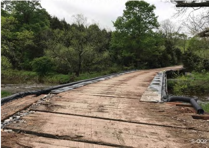
Figure 1: Stream S-QQ2 – Controls in place and functioning properly around stream crossing. (Sinking Creek) BRG: 178°S (T) LAT: 37.333126 LON: -80.431150 ±541ft ALT: 2008ft
